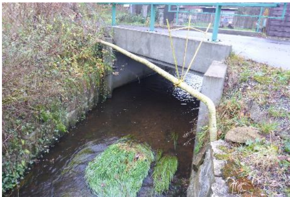
Obr. 170. Most M-06 v ř.km 1,303 (-731237, -942615)
