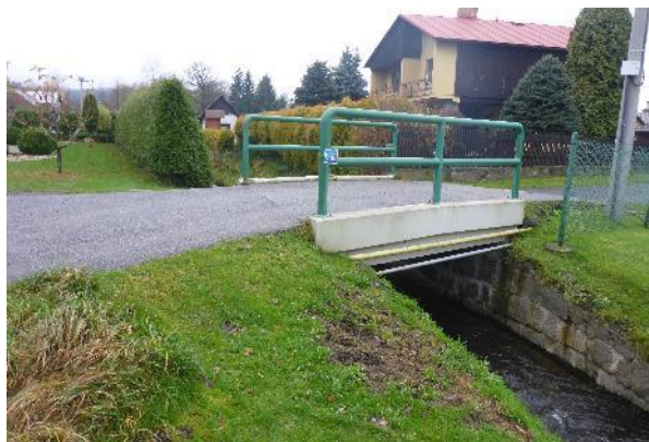
Obr. 165. Most M-10 v ř.km 0,857 (-731439, -942904)
