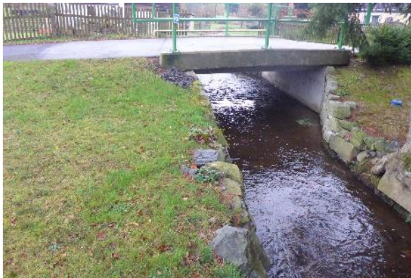
Obr. 168. Most M-08 v ř.km 1,157 (-731247, -942729)
