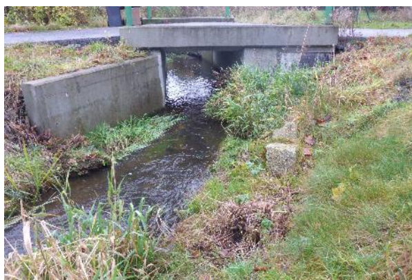
Obr. 179. Most M-02 v ř.km 1,948 (-730935, -942049)
