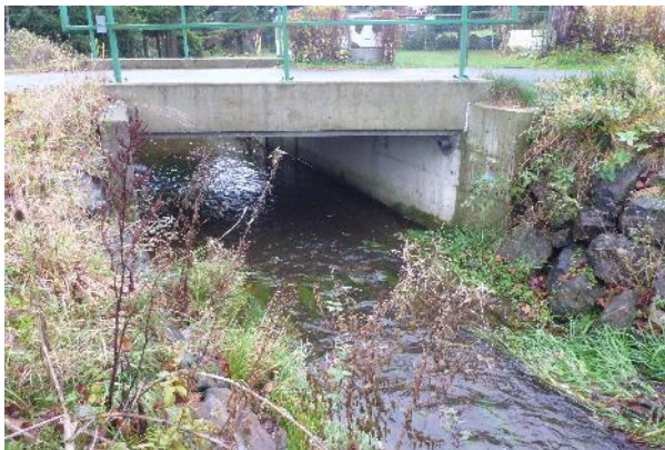
Obr. 172. Most M-05 v ř.km 1,479 (-731174, -942436)
